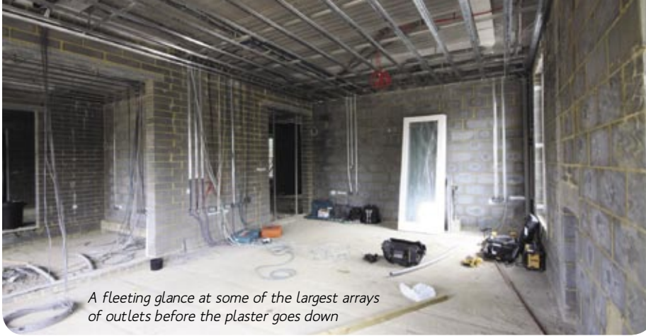
Hanging wire routing is simplified in this area by a joinery feature partitioning one room from another which serves to ease the cable run
