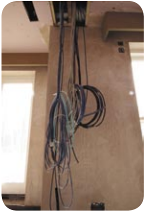
Hanging wire routing is simplified in this area by a joinery feature partitioning one room from another which serves to ease the cable run
